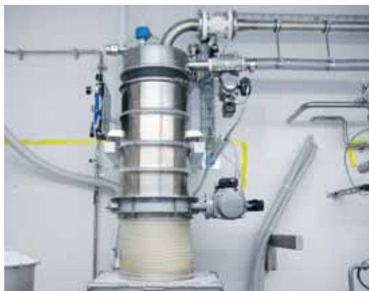
Vacuum conveyor for sugar
