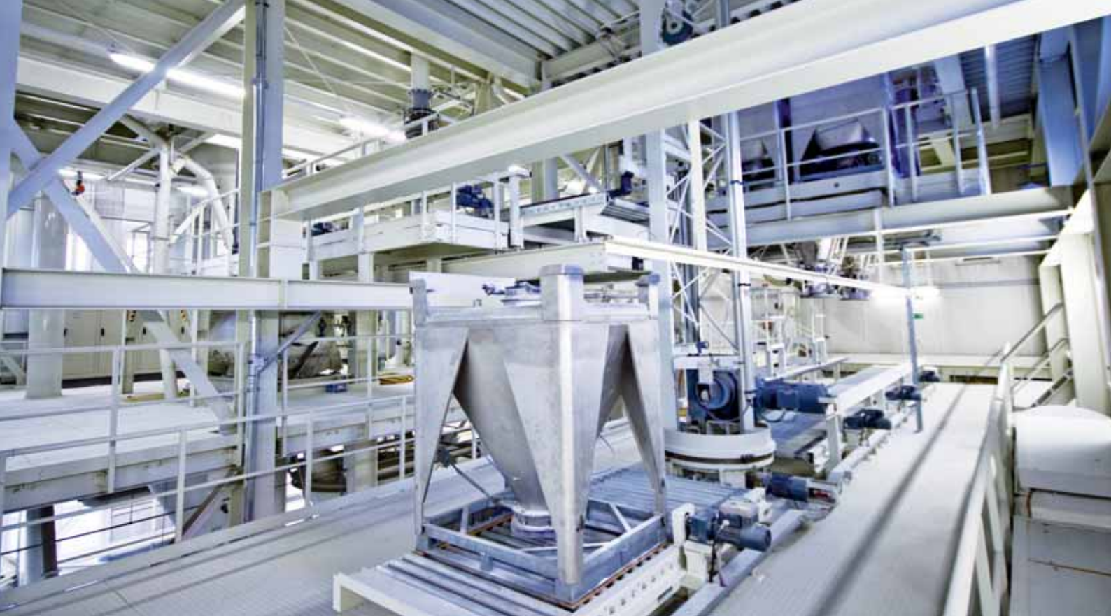
Batchbin loading equipment
