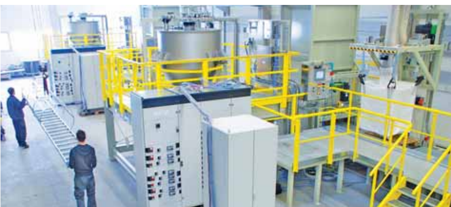
Setting up plant for works approval
