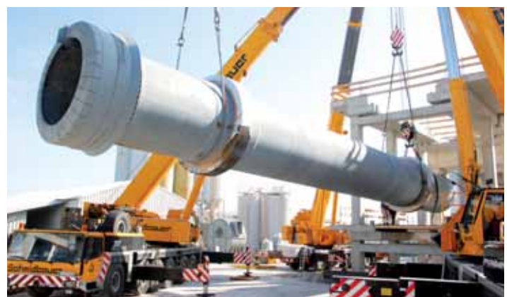
Fitting a kaolin cooler
