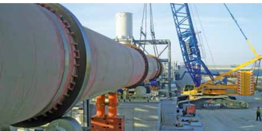
Installing a rotary kiln
