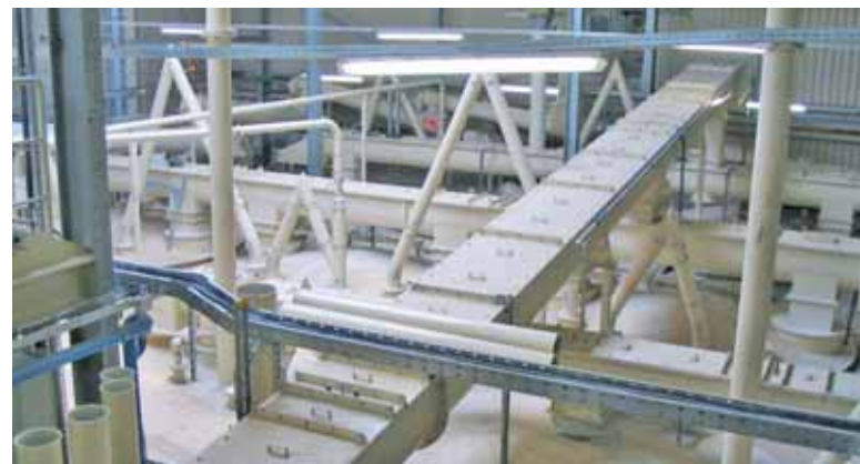
Building materials being conveyed with trough screw conveyors
